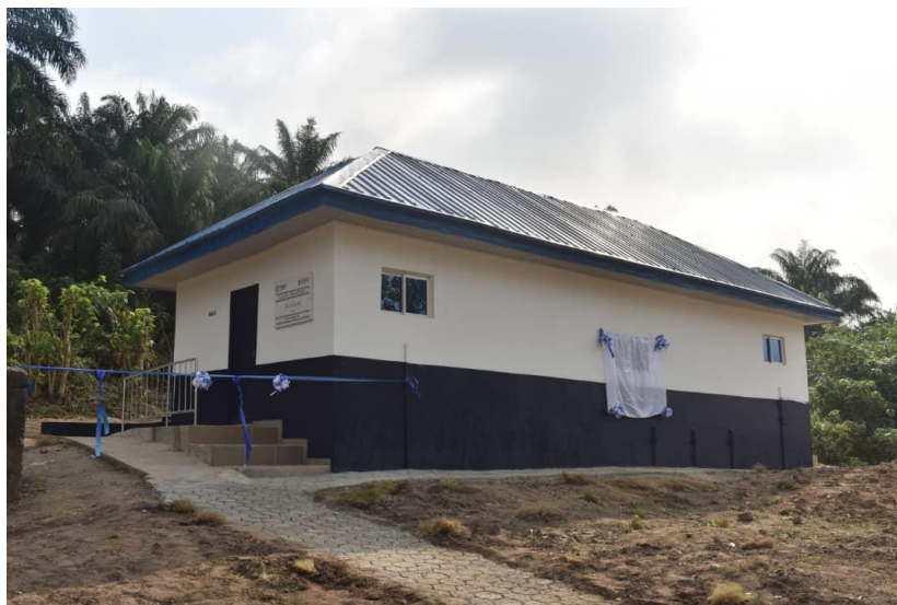
Photo 6: New sanitation facility constructed by WADA Project at Government Secondary School, Ndon Nwong, Odukpani LGA, Cross River State on the day of project commissioning, December 2018.
